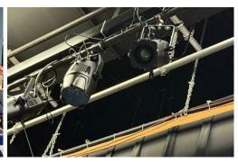
Coverage for the third and fourth stage layers comes from the KL PROFILE COMPACT, a smaller ellipsoidal with a 25° to 50° zoom and framing features. "A valued feature of this fixture is its ability to accommodate gobos, making it the ideal addition for this project," Dunlap added.
